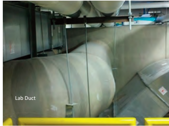
Minneapolis Water Plant, Ammonia Addition Duct, Lab Duct
